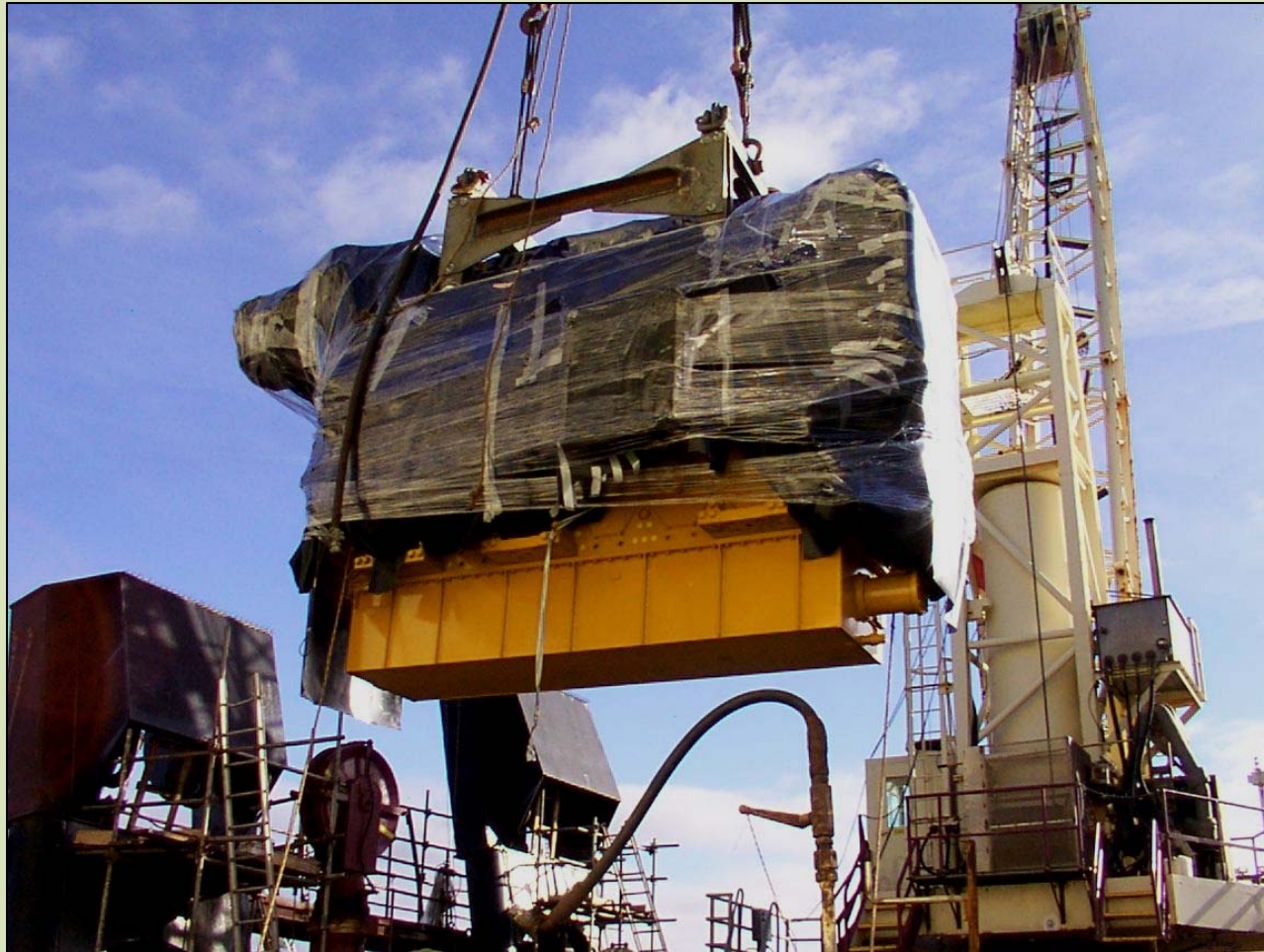
New Tier II CAT Engine being rigged into the engine room
